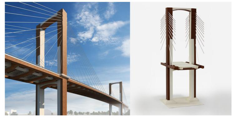
The Centenario Bridge in Seville shares a structural typology and cable technology with the Fernando Reigh Bridge in Alcoy. Both bridges of the State Highway Network employed the cable technique available at the time of their construction: prestressed strands embedded in cement grout confined in a black polyethylene outer sheath. The only difference between them being that a second outer sheath with a white finish was placed on the Centenary Bridge.
